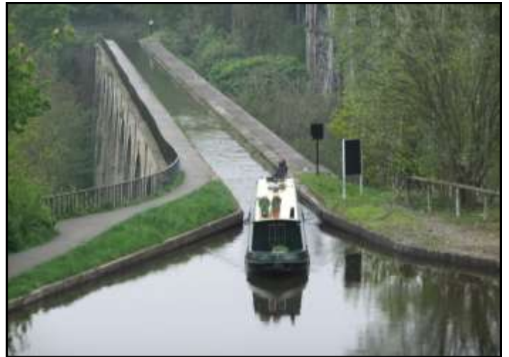
Marian Lovegrove's Narrow Boat Brimble as she crossed over the Chirk Aqueduct.
