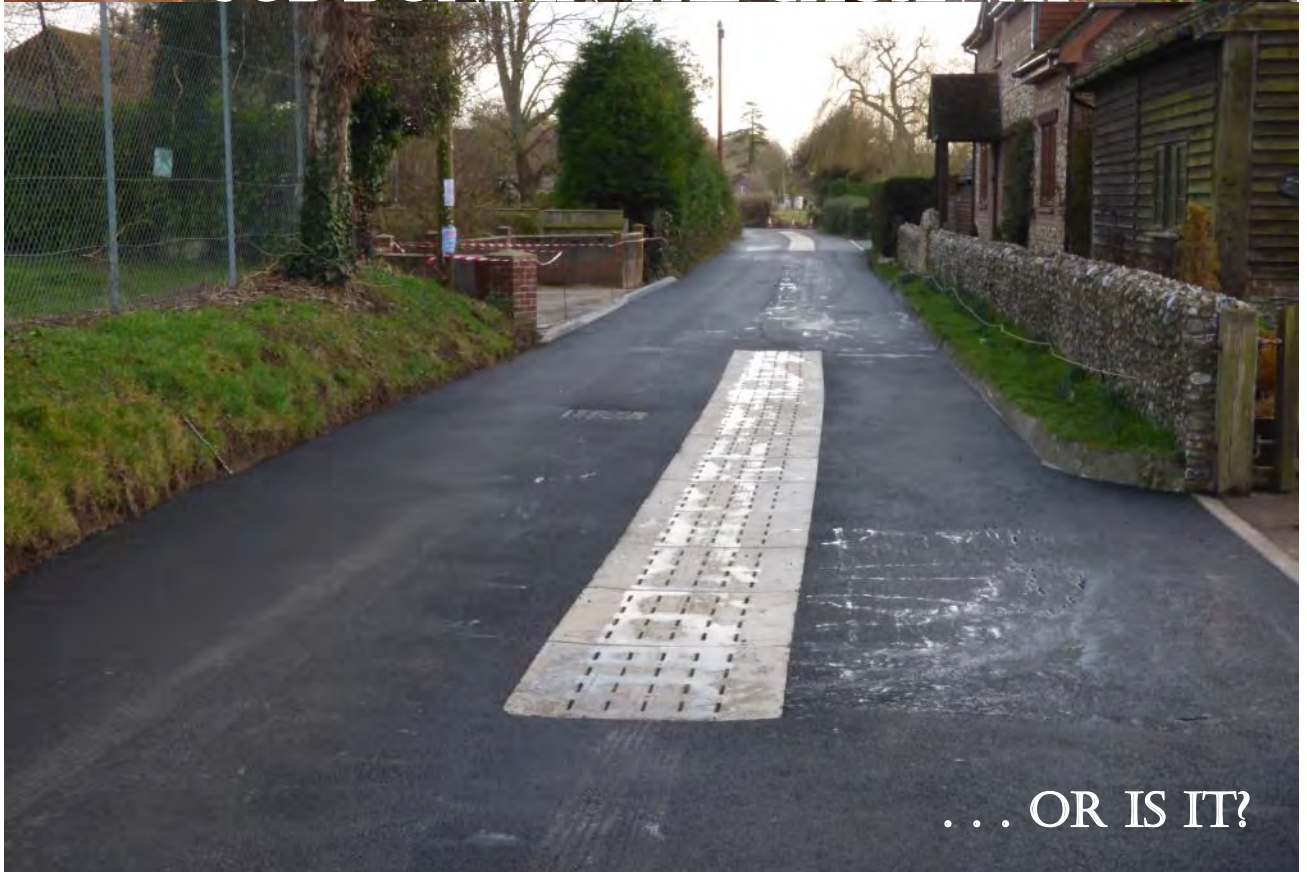
JOB DONE IN THE CAUSEWAY
