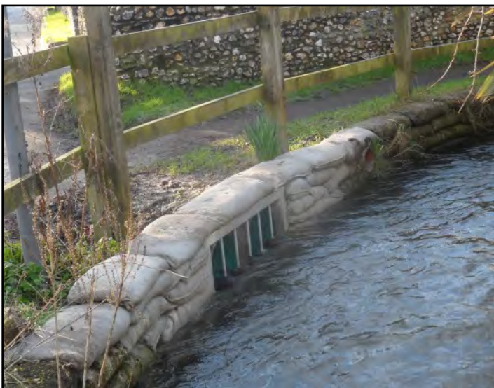
The overflow in The Causeway seems to be working.
