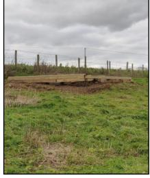
Although it hasn't been exactly goat shed building weather, our hardy band of volunteers has been undeterred. The ground has been dug away at the site of the new shed, and a sturdy base of reclaimed railway sleepers installed with a basic framework for the floor. During the last week or so, the uprights have been cut correctly (remembering before to measure twice of
